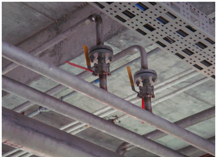
Branches tie-in from above into a main header
